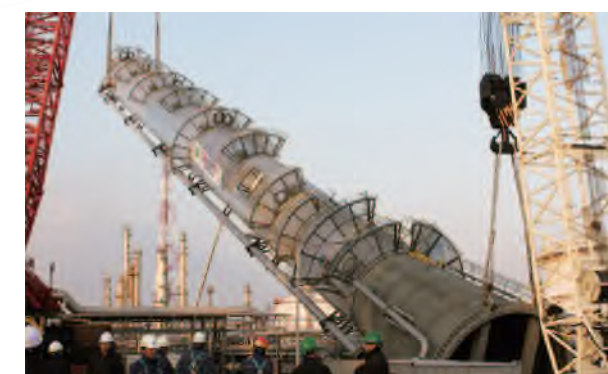
Propylene Rectifier (Full Dressed, SA516-70N) • Client : Korea Petrochemical Ind. Co., Ltd./ Korea (2016) • Size(mm) : 39T X ID 4,800 X L 87,510 / 715.9 Ton
